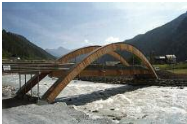
Brücke San Niclò bei Strada, CH. Bridge San Niclò near Strada, CH. Quelle/source: Andrea Bernasconi, HES-SO Yverdon/ LIGNUM.
