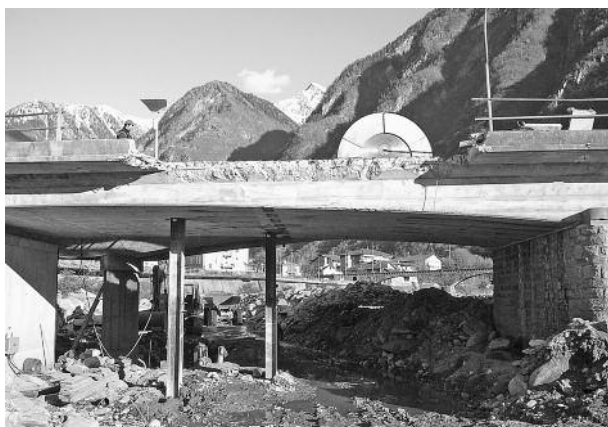
Sägen der vier 4.70 x 1.00 m grossen Segmente. Cutting of the four sections with a size of 4.70 x 1.00 m.
