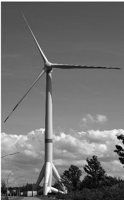
Prototyp einer Multibrid M5000 Offshore-Windenergieanlage. Prototype of a Multibrid M5000 offshore wind energy converter.
