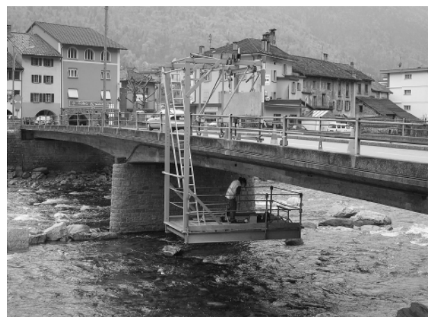
Installation der Sensoren. Installation of the sensors.
