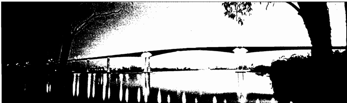
Brisbane's Gateway Bridge, was designed and detailed using many of the concepts and methods described in this report.
