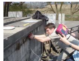
Investigated Concrete Element while conducting the Electrical Resistivity Test
