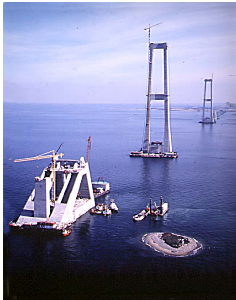
Great Belt Bridge under Construction
