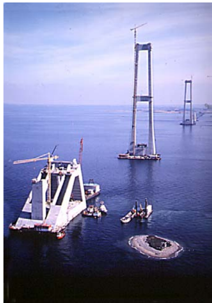
Great Belt Bridge under Construction
