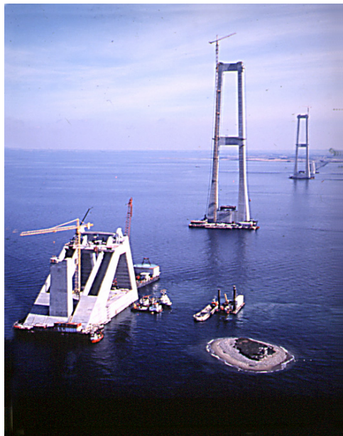
Great Belt Bridge under Construction
