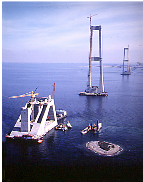
Great Belt Bridge under Construction
