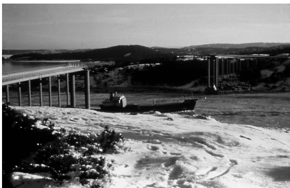
Figure 1.8: Tjörn bridge after collision with a ship in January 1980.
