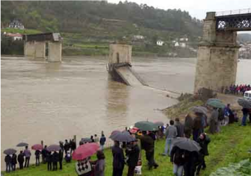
Figure 4.12: Failure of a roadway bridge due to scour, Portugal, 2001.
