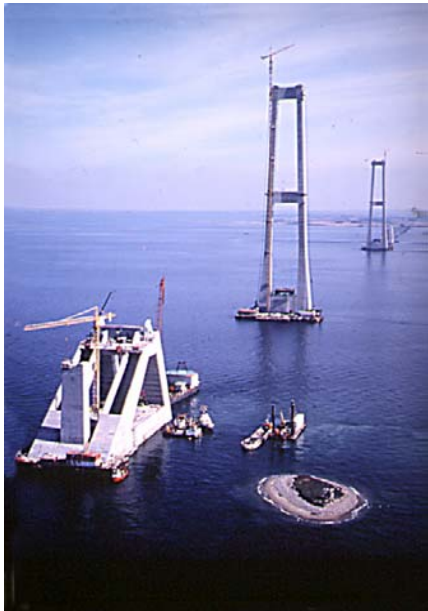
Great Belt Bridge under Construction
