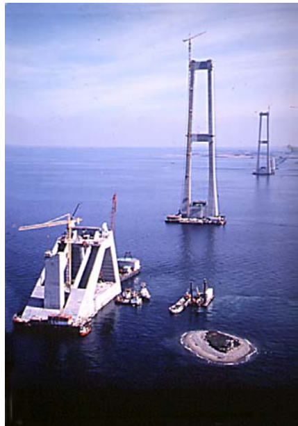
Great Belt Bridge under Construction
