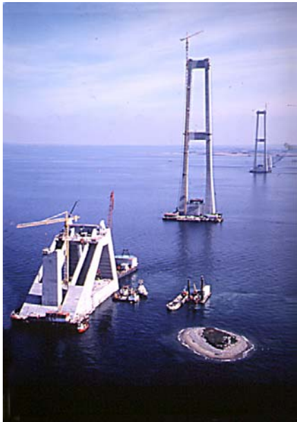
Great Belt Bridge under Construction
