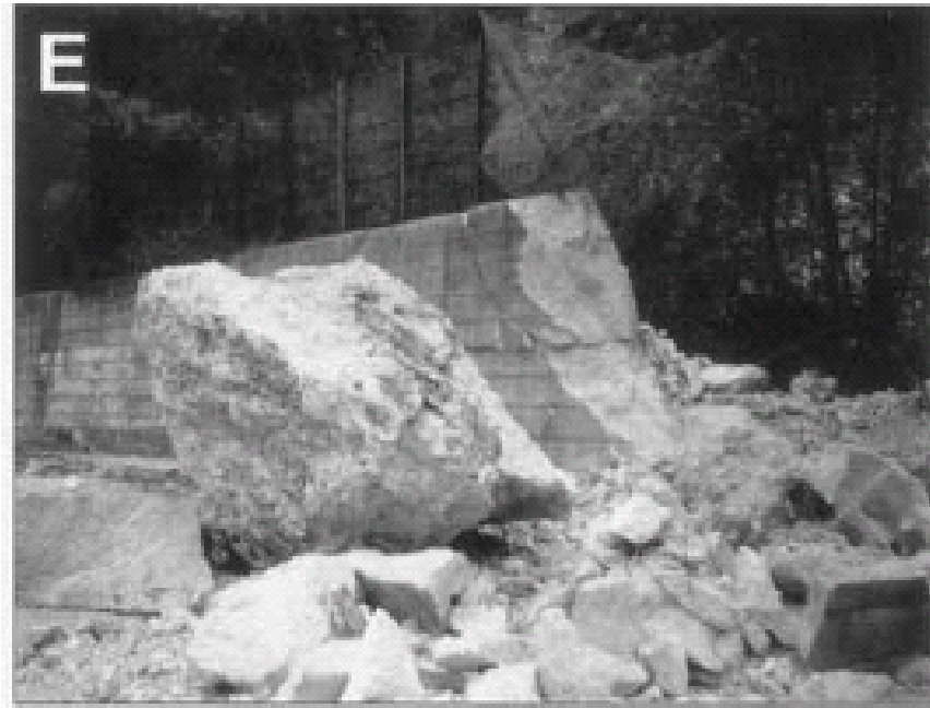
Concrete retaining walls
