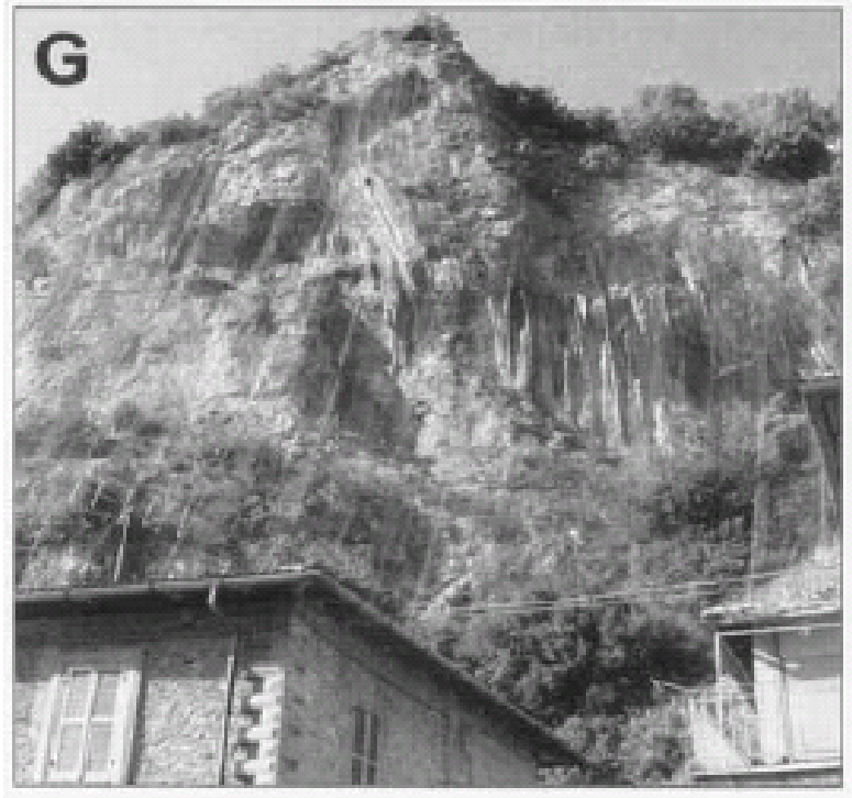
Passive revetment nets
