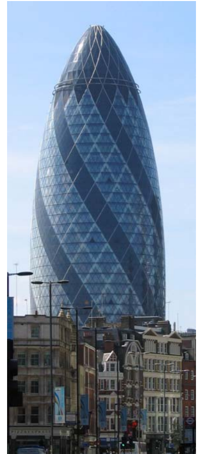
Swiss Re "Gherkin", with a lattice shell by Norman Foster and Ken Shuttleworth, London.
